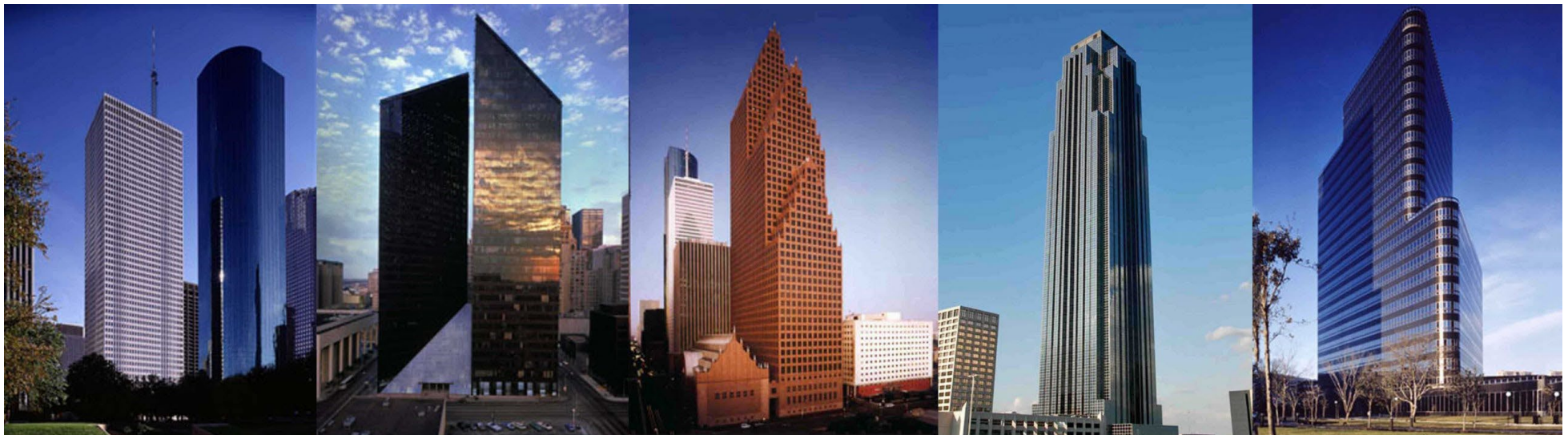
One Shell Plaza: Pennzoil Place: Bank of America Center; Williams Tower; One Post Oak Central
